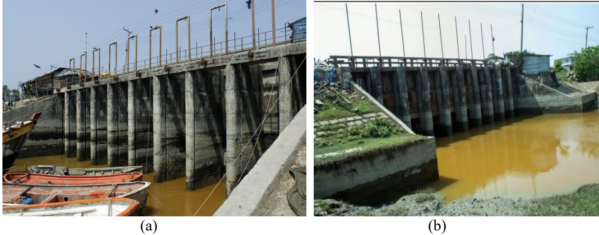
Figure 5.2 Sluice gate of the polder 61/1 in Kumira [a. sea facing side; b. polder facing side of the sluice gate.]
